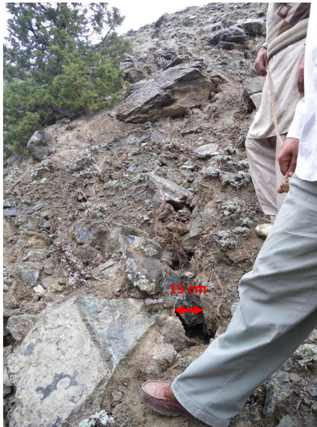
Figure 7: Tension crack on the right side of the landslide with a gap of 15cm.
