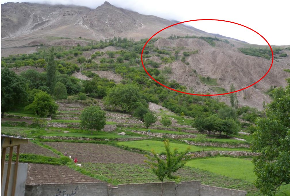
Figure 21: Upper Nagar landslide inside the red circle.
