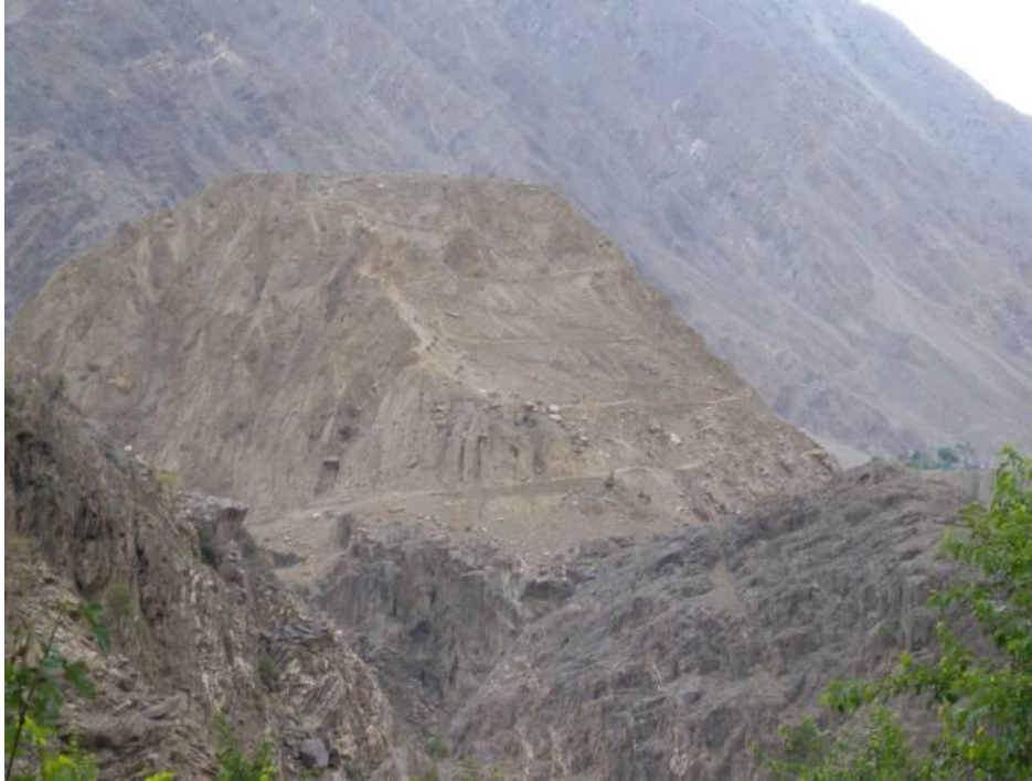
Figure 1: Road to Khaltaro and Dasso villages built on alluvial terrace. The instability is very high as the danger while running this road.
