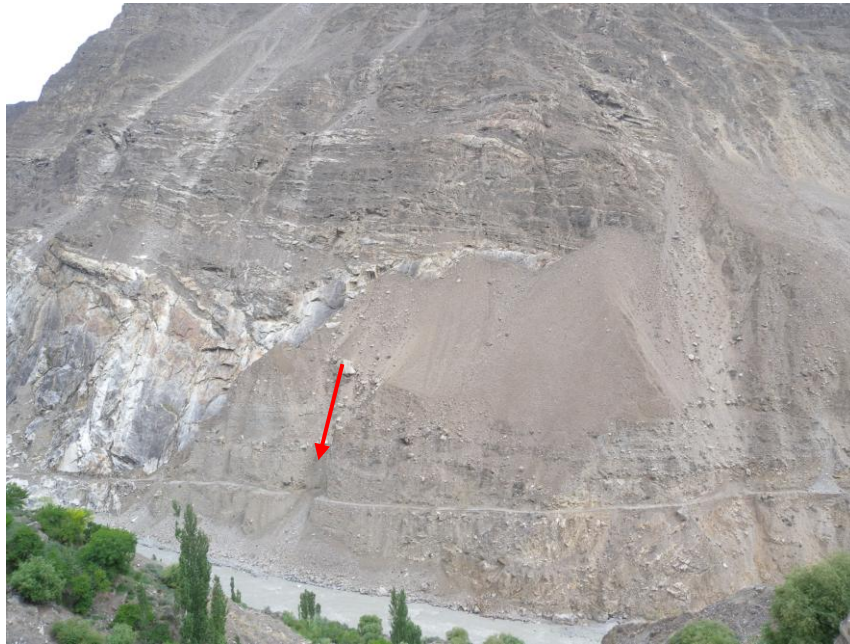
Figure 20: Old road to Nagar interrupted in several points by landslides. Red arrow indicates one of the interrupted points.
