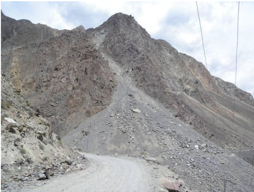
Figure 15: An active landslide on the road to Bagrot valley.
