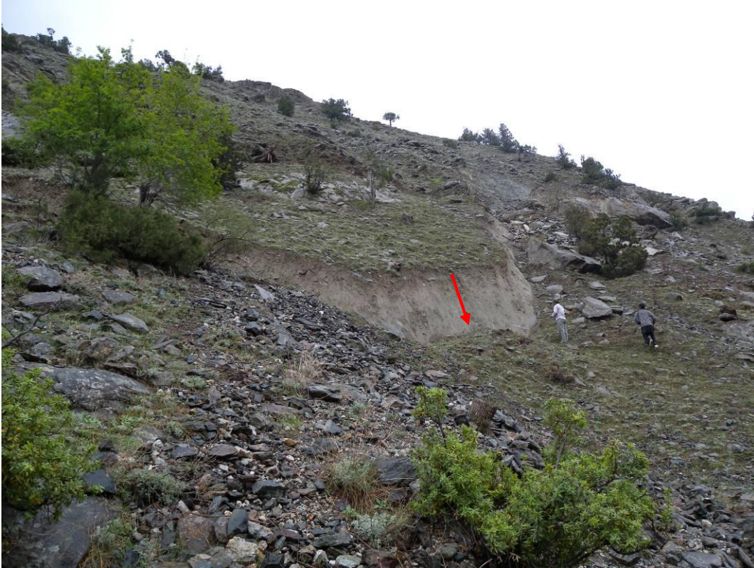
Figure 5: Khaltaro landslide, the main scarp is clearly visible; its high is approximately 4m.
